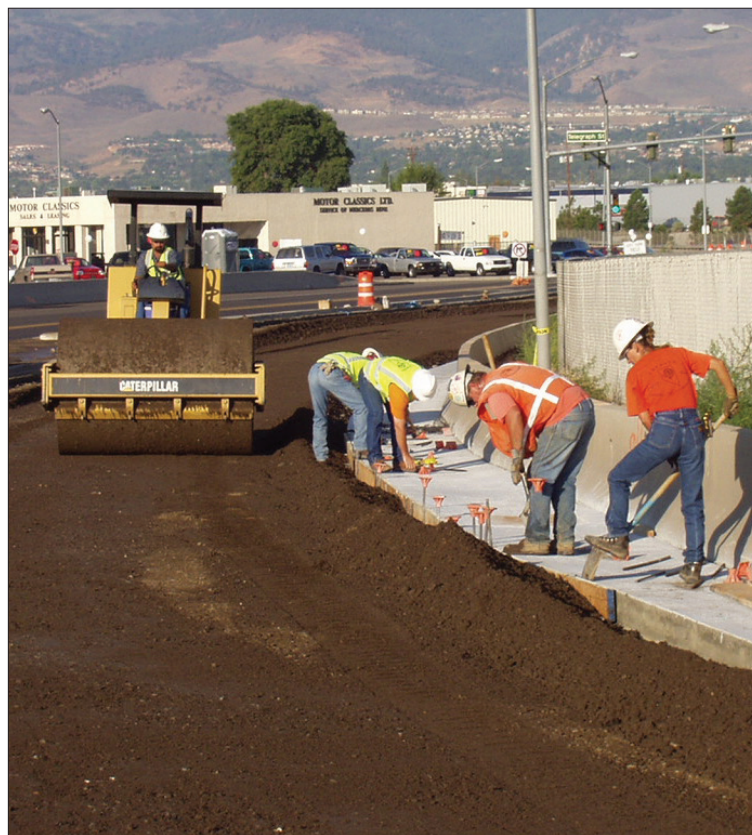
Maintenance on roadway
