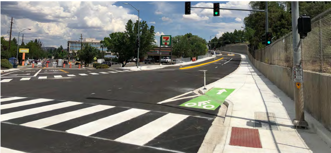
Keystone Avenue & California Avenue Intersection.
