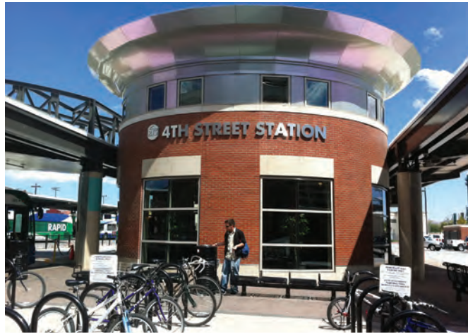
Bike racks at RTC 4TH STREET STATION.
