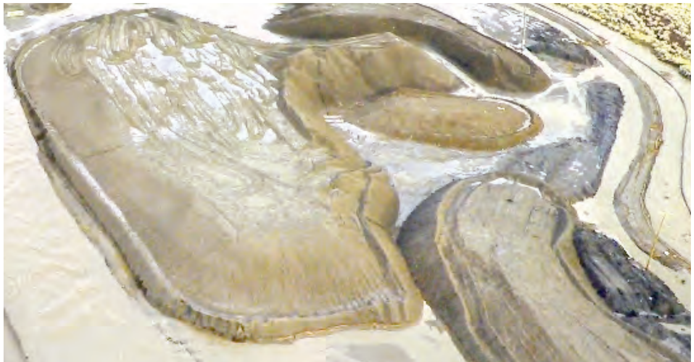
The SouthEast Connector is designed to store stormwater runoff and reduce flooding in nearby areas, as demonstrated during the 2017 flood events.
