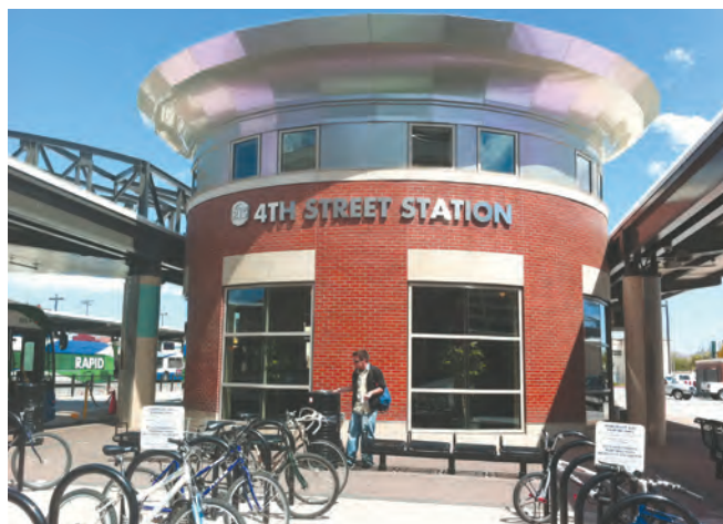
Bike racks at RTC 4TH STREET STATION.
