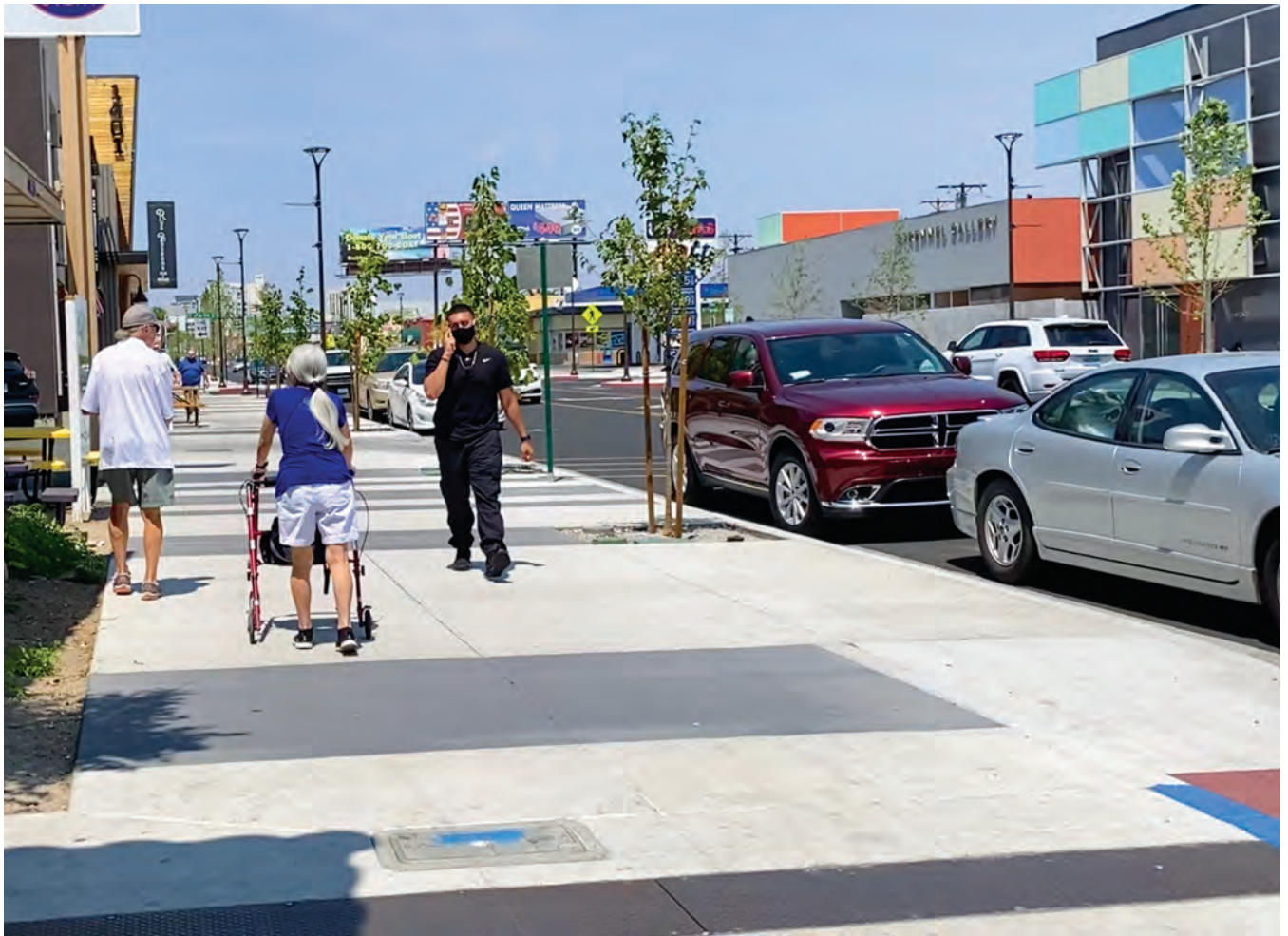
Virginia Street: Safety improvements, like widened sidewalks, provide ample space for social distancing during the 2020 COVID-19 pandemic.
