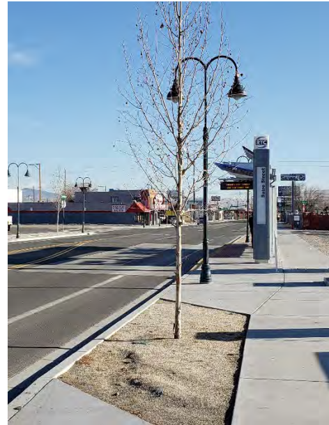
Photo 3. Sutro Street BRT Station
