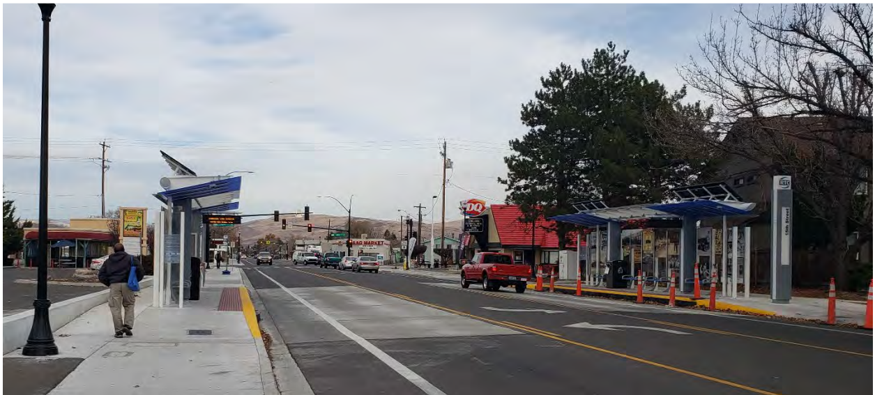
Photo 1. Prater Way at 15 th Street (location #2) with newly constructed RTC RAPID Stations.
