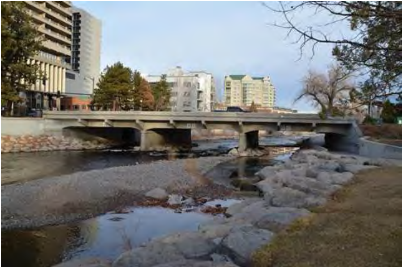
Existing Three Span (Two Pier) North Bridge
