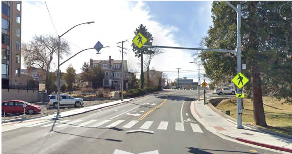
Figure 7. Existing Crosswalk and overhead flashing signage along south side of Island Avenue / Arlington Avenue intersection.
