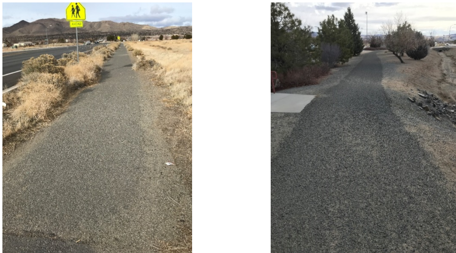
Figure 5.15: Existing Shared Use Path North side of Eagle Canyon Drive
