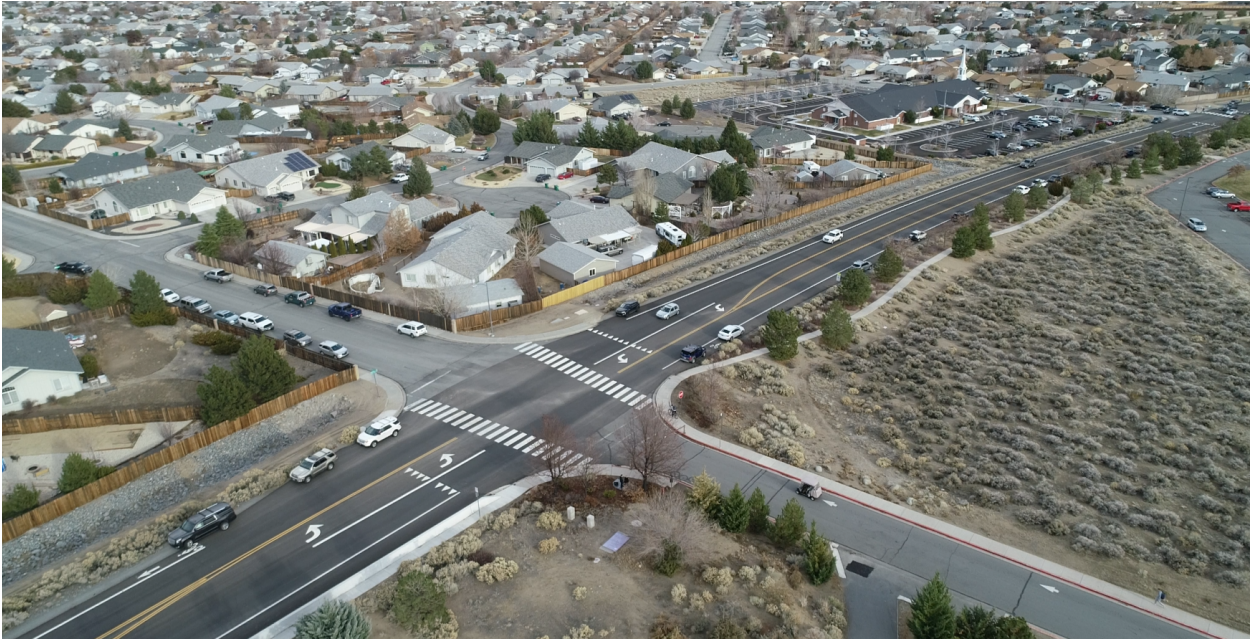
Figure 5.12: Goldeneye Parkway Crosswalks Drone Footage
