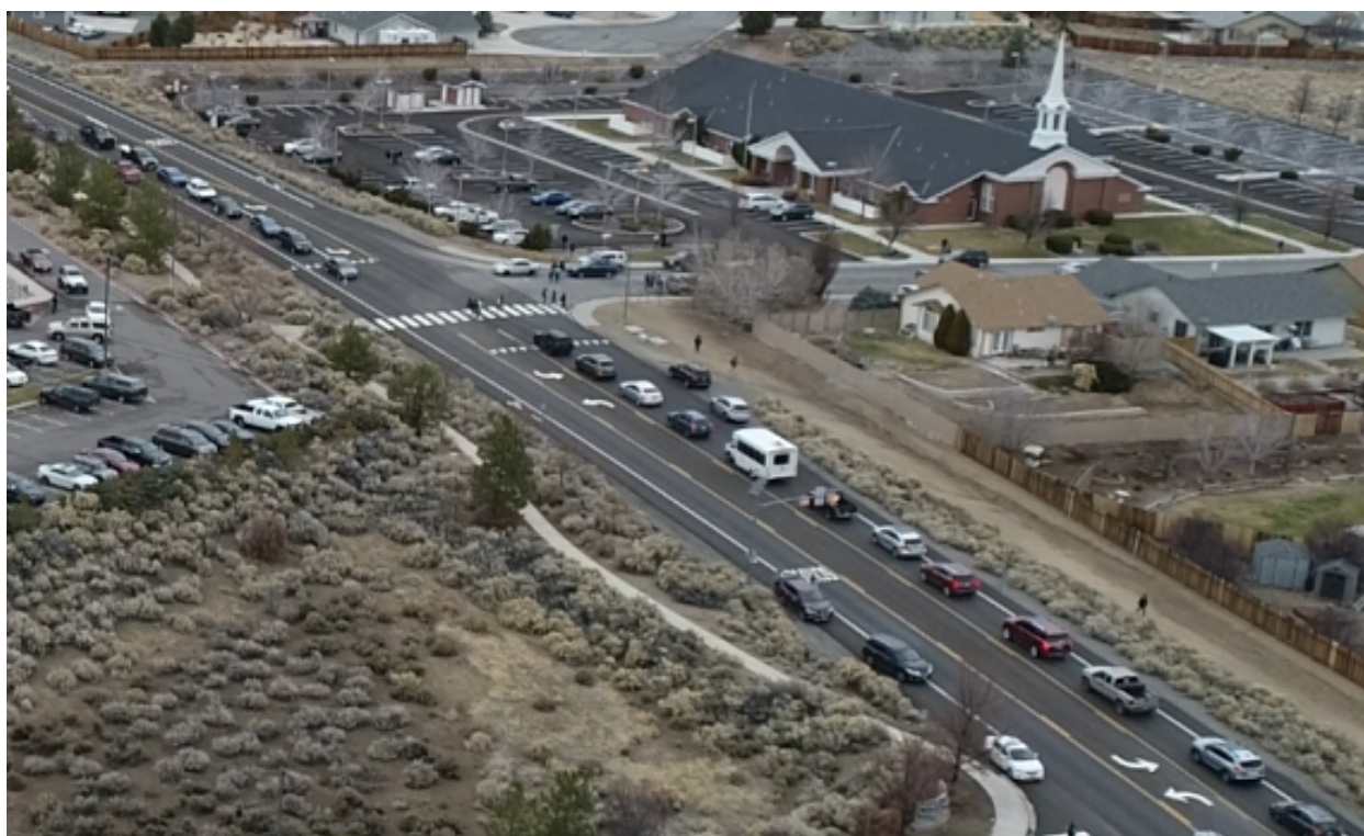
Figure 5.11: Spanish Springs High School – Mercedes Drive Crosswalk Drone Footage
