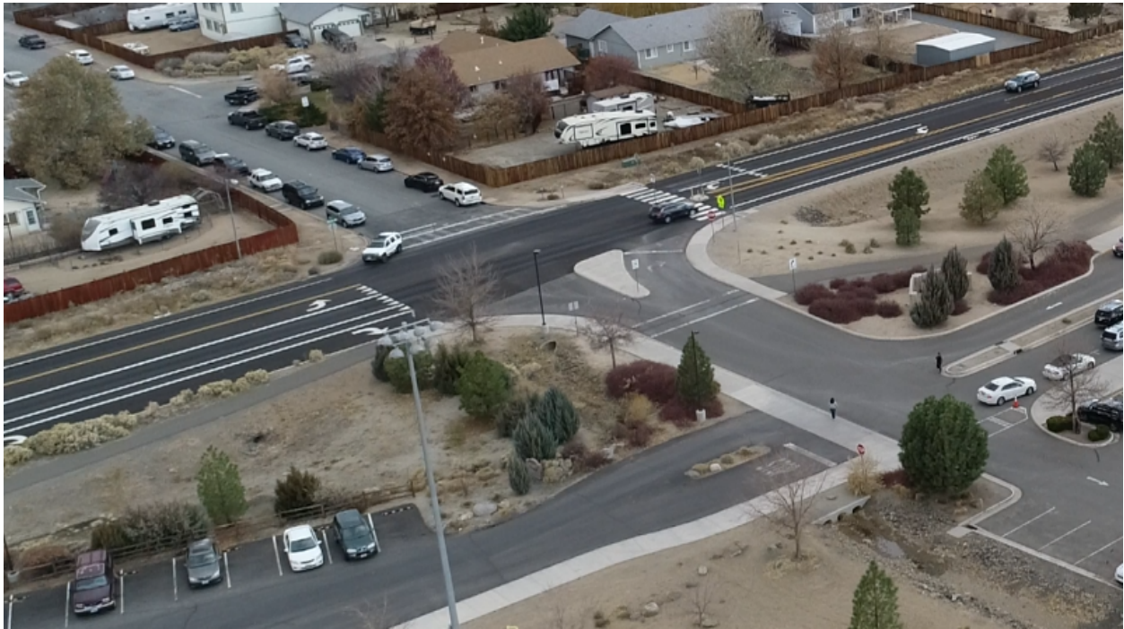
Figure 5.9: Drone Footage – Missy Drive & Eagle Canyon Drive Crosswalk
