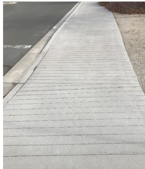
Figure 5.22: Non ADA Compliant Ramp @ Shaw Middle School
