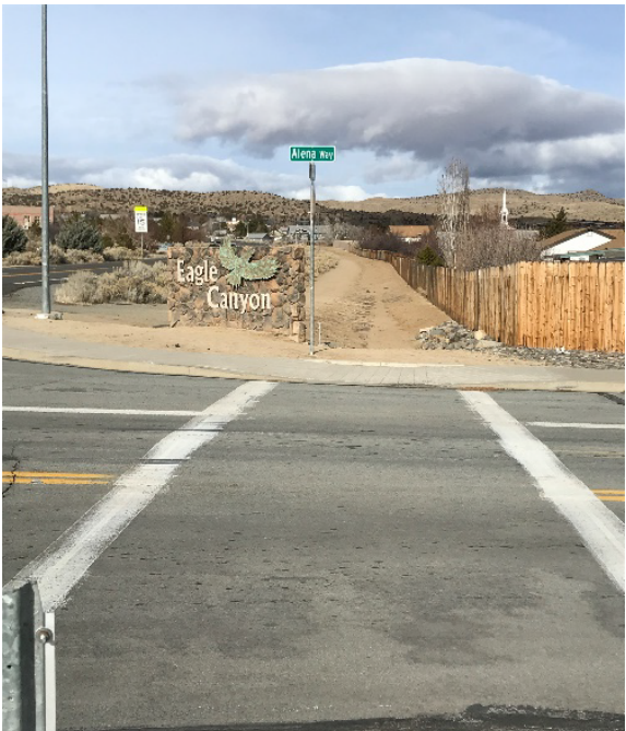
Figure 5.16: Alena Way Southbound Approach Crosswalk Striping
