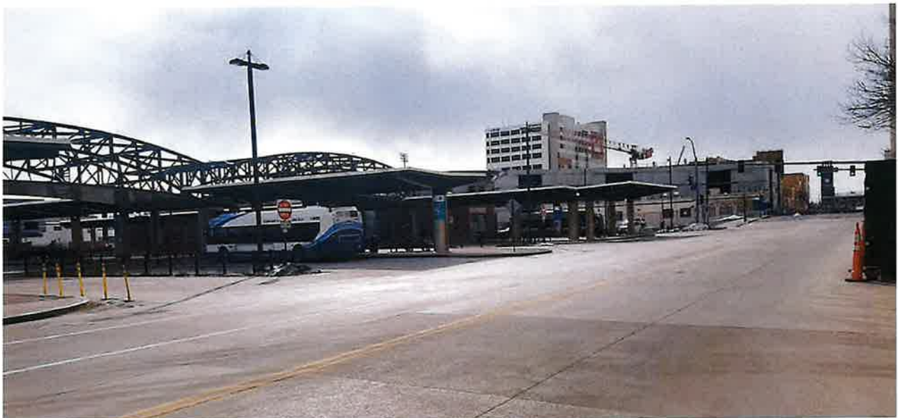
Bus bays at the RTC 4th Street Station reduce potential for maintaining physical separation between cyclists and vehicles
