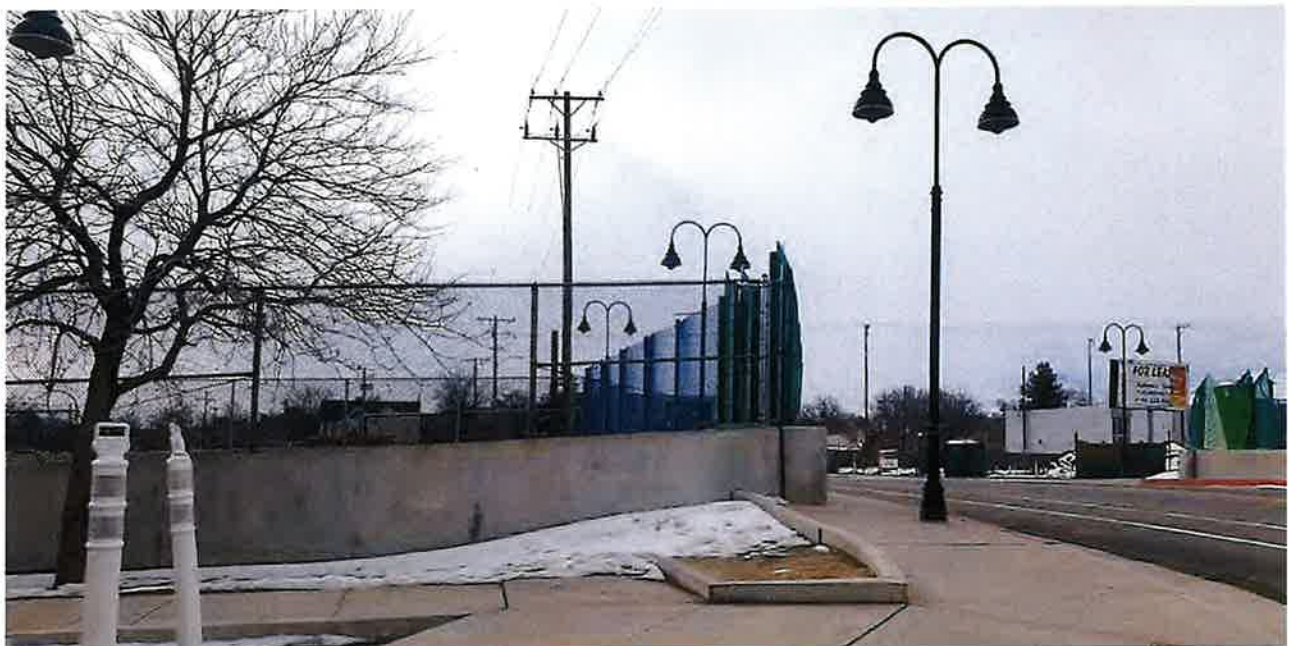
The existing train trench wall presents a potential sight distance issue for bicyclists and pedestrians crossing major streets
