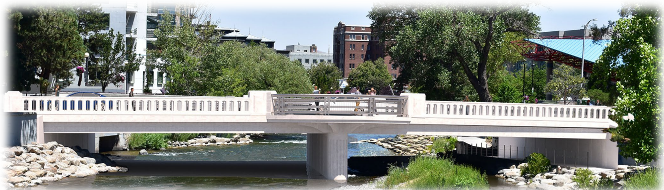
Figure 6. Hybrid Concrete with Metal Railing at Overlook
