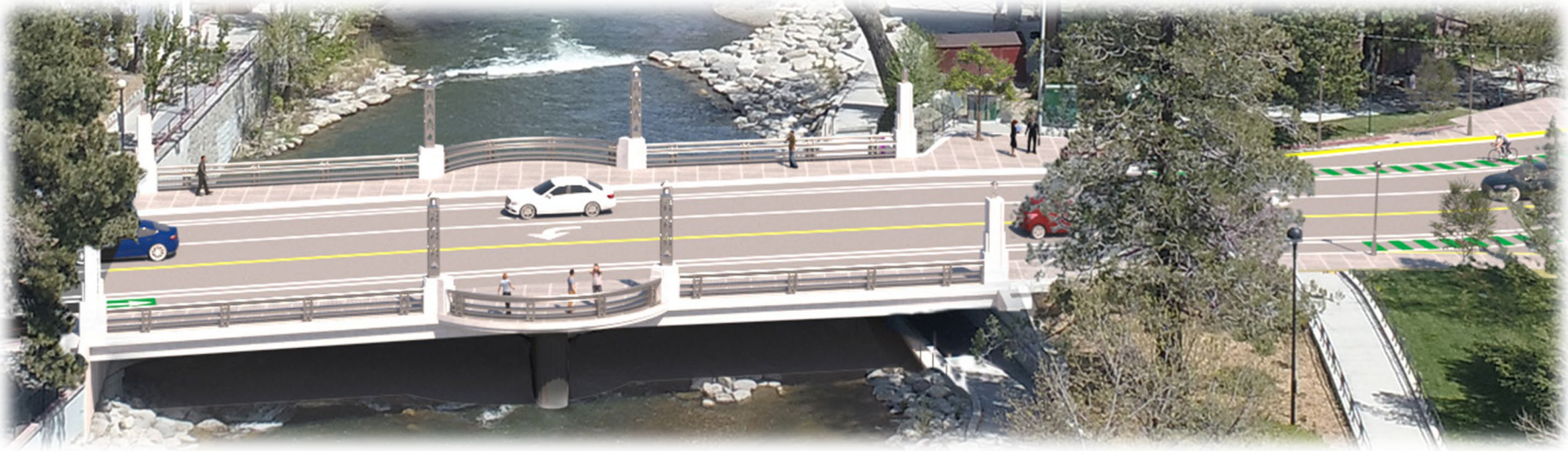
Figure 13. North Bridge Blow up
