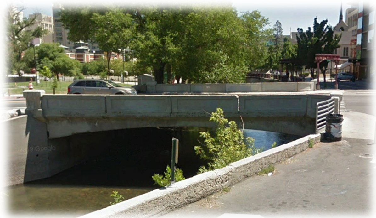
Figure 3. Existing South Bridge
