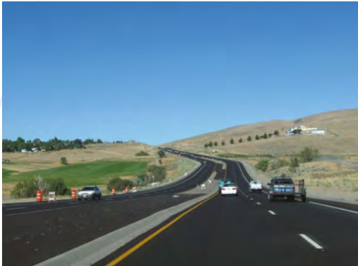
^ McCarran Boulevard, adjacent to San Rafael Regional Park.
