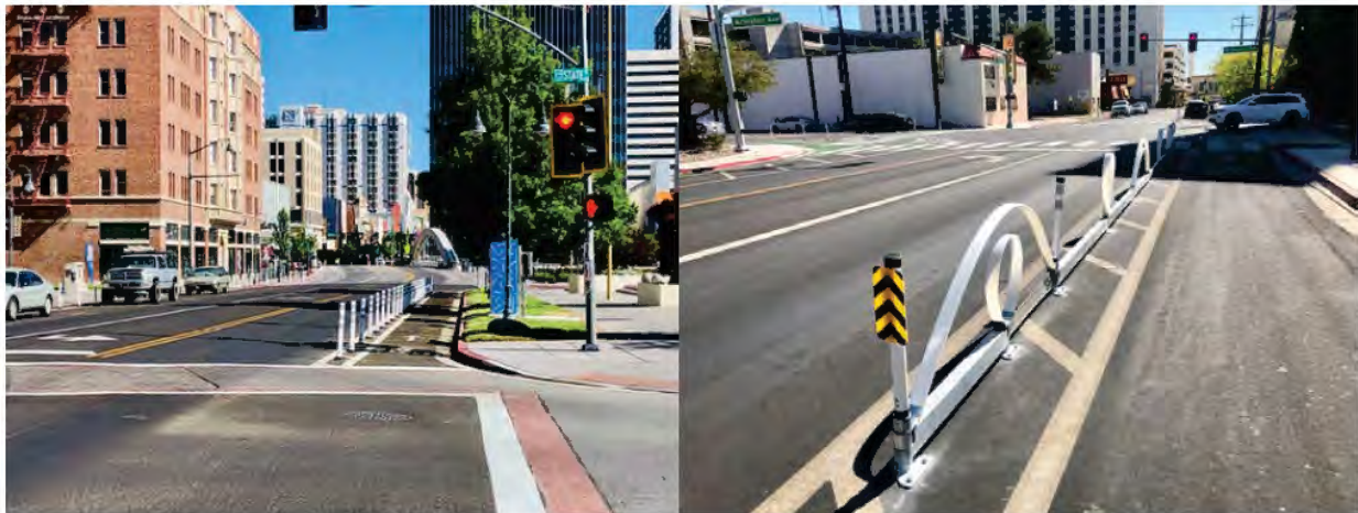
Figure 2-2 - (Left) Delineated buffered micromobility lane, (Right) Artistic bike rail.
