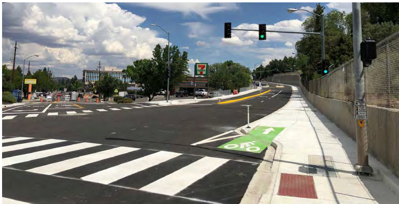
Keystone Avenue & California Avenue Intersection.
