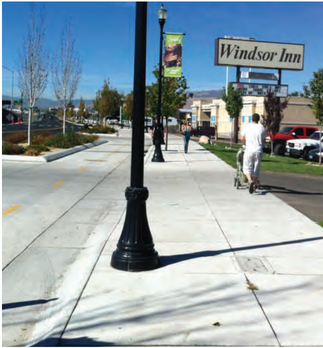
Victorian Avenue in Sparks. The project included the addition of a cycle track, wider sidewalks, and improved bus stops.
