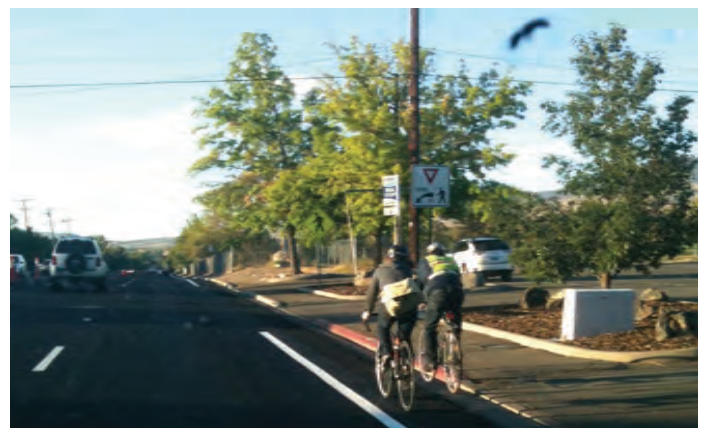
Bicyclists and joggers on Plumas Street after Complete Street project
