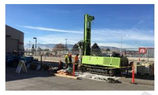
VILLANOVA MONITORING WELLS PROJECT IS UNDERWAY - The Underground Storage Tank monitoring wells are being installed at 2050 Villanova as required by Nevada Division of Environmental Protection (NDEP). These wells will be used to monitor soil contamination from a previous diesel spill that was mitigated in 2016.
