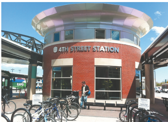
Bike racks at RTC 4TH STREET STATION.
