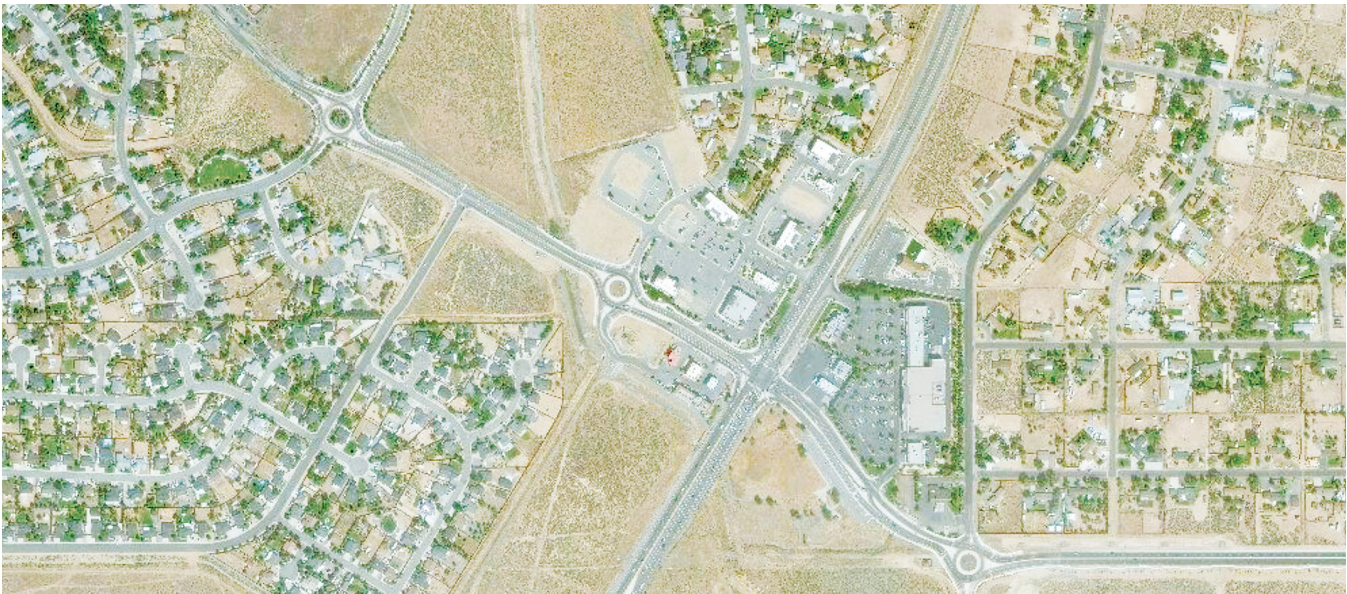
Roundabouts along Eagle Canyon Drive and La Posada Drive.
