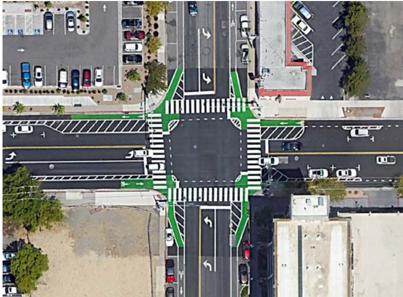
Figure 2-6 - Protected Intersection at 5th Street and Arlington Avenue.
