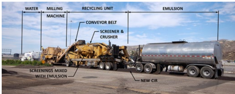
Figure 23. Cold in-place recycling train components.
