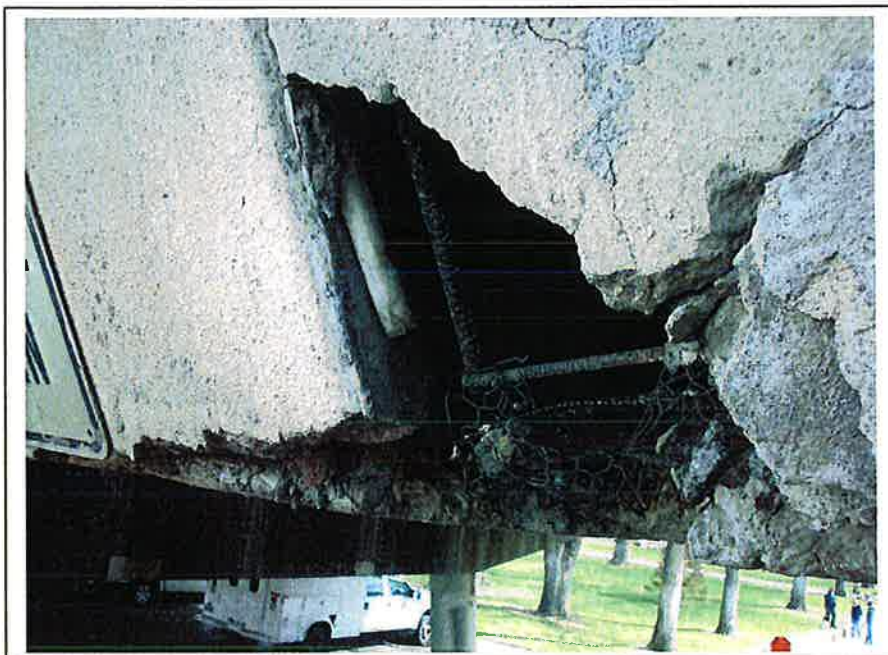
Photo 7 - Span 3 Impact Damage
