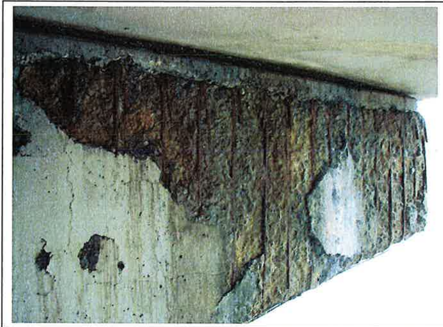
Photo 9 – Deteriorated/Spalling Concrete at West End of Pier 3 Cap
