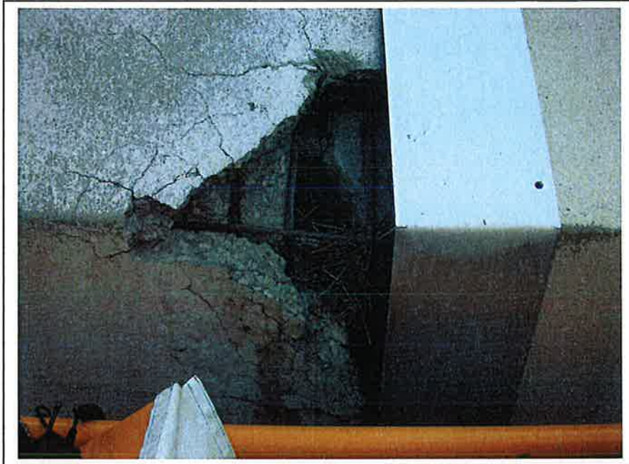
Photo 5 - Spall at Joint 3 in Span 2
