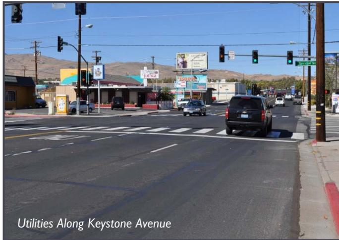
A field inventory of visible utilities within the right-of-way was conducted for the corridor. This preliminary survey identified locations of utility poles, signal poles, pedestrian push buttons, power lines, communication and pull boxes, and other visible utilities. Detailed survey sheets are provided in Appendix J.
