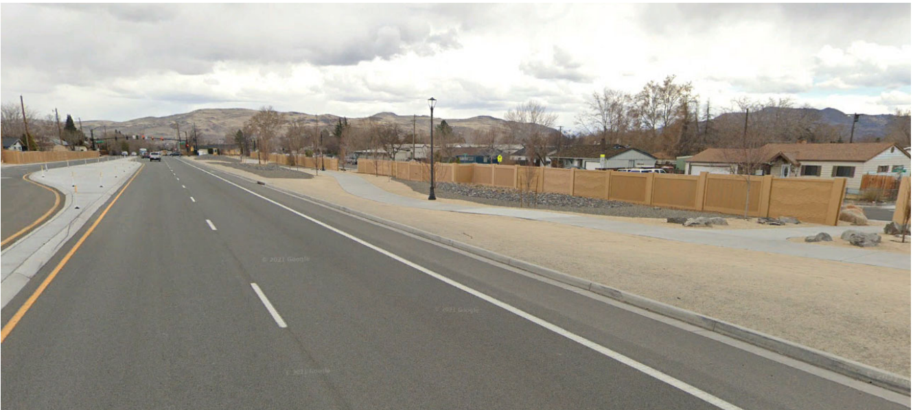
Image: Detached sidewalks with lighting along northeastern McCarran Boulevard
