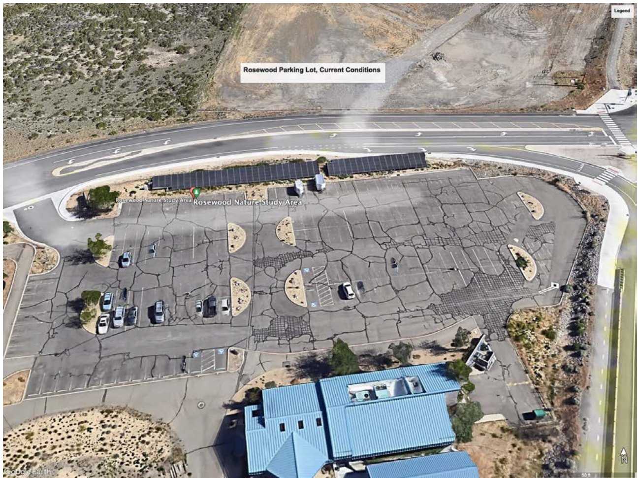
Rosewood Parking Lot: Current Conditions
