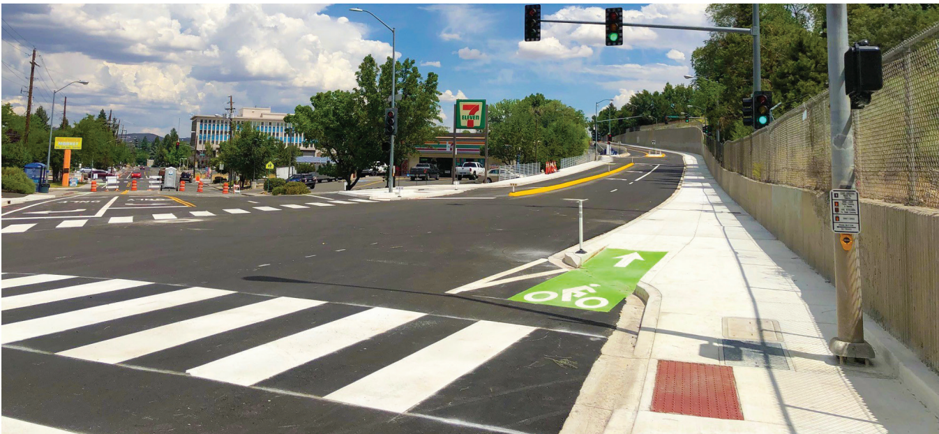
Keystone Avenue & California Avenue Intersection.
