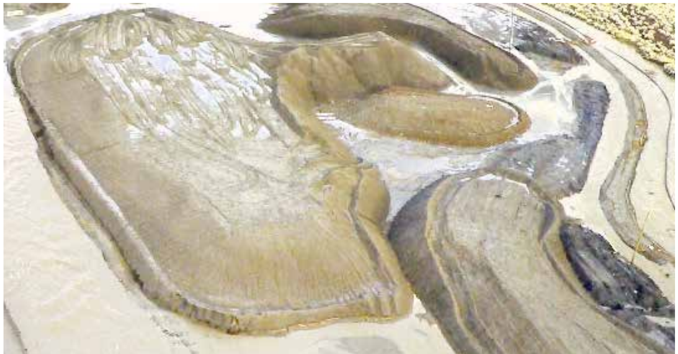
The SouthEast Connector is designed to store stormwater runoff and reduce flooding in nearby areas, as demonstrated during the 2017 flood events.
