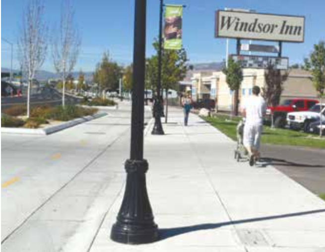
Victorian Avenue in Sparks. The project included the addition of a cycle track, wider sidewalks, and improved bus stops.
