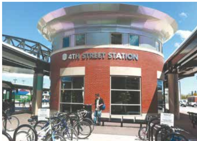
Bike racks at RTC 4TH STREET STATION.
