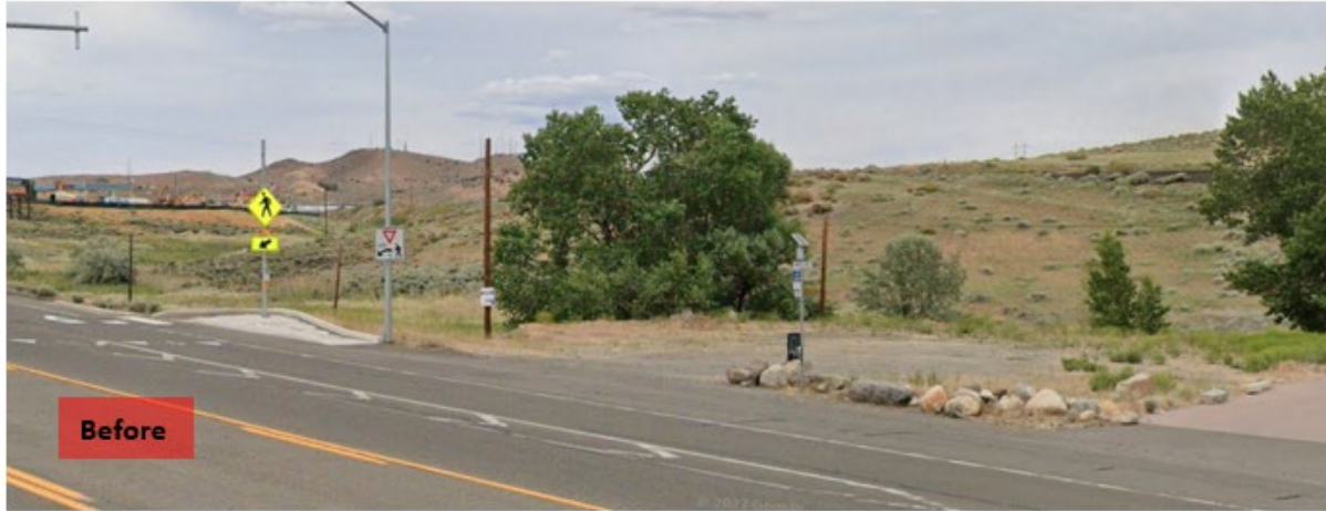
BSL 346 N Virginia St before Talus northbound – Route 7
