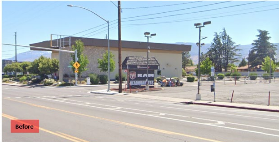
BSL 445 Kietzke Ln and Roberts St southbound – Route 9
