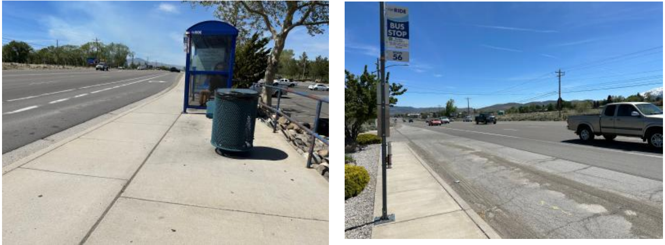
Figure10 - Existing Bus Stops on S Virginia Street for Route 56 & the Regional Connector
