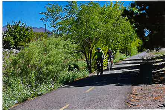
The Sparks Blvd shared-use path provides a low-stress environment for bicyclists traveling along this arterial roadway.
