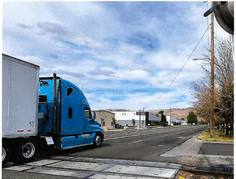
Railroad crossing on Glendale Avenue
