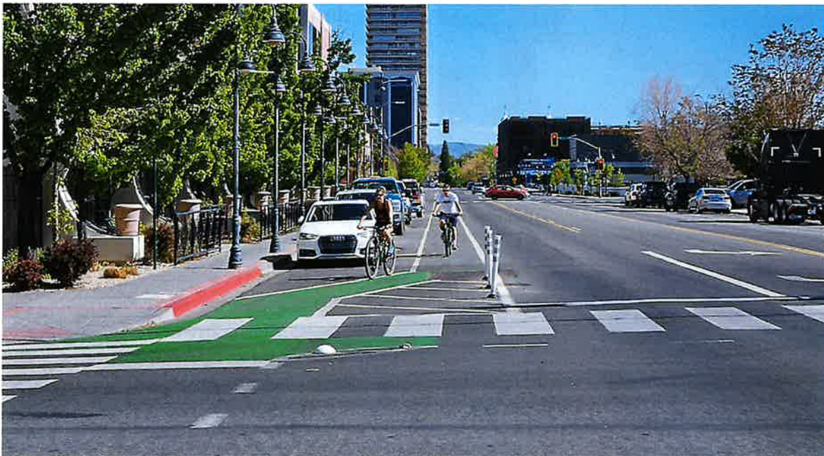
Providing greater separation for bicyclists at intersections helps bicyclists navigate through these junctions.
