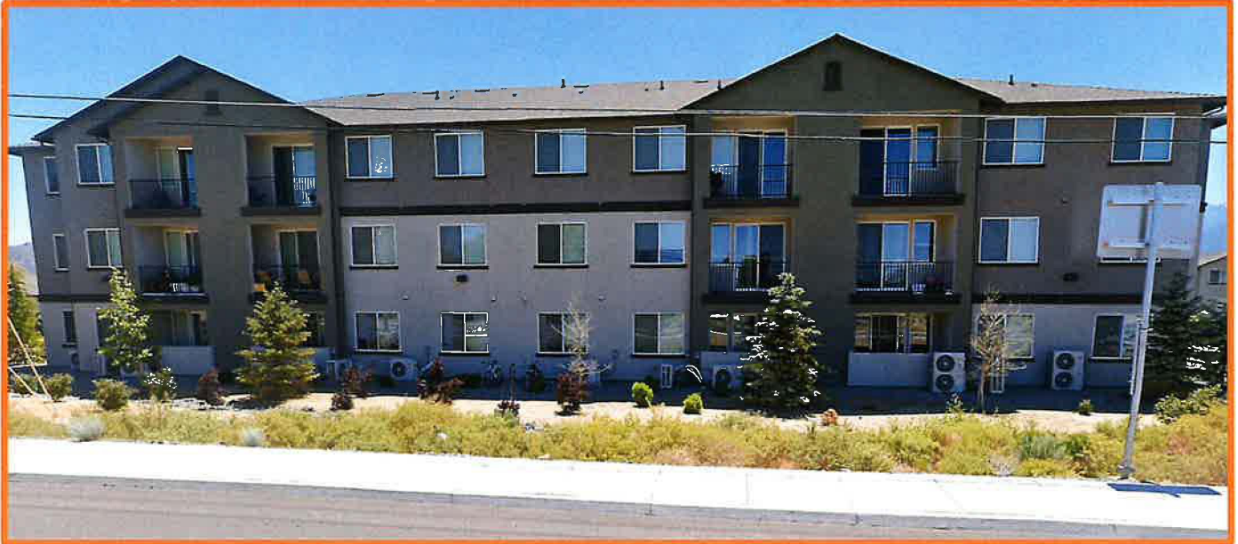
Steamboat Apartments Located Along Geiger Grade (SR 341)
