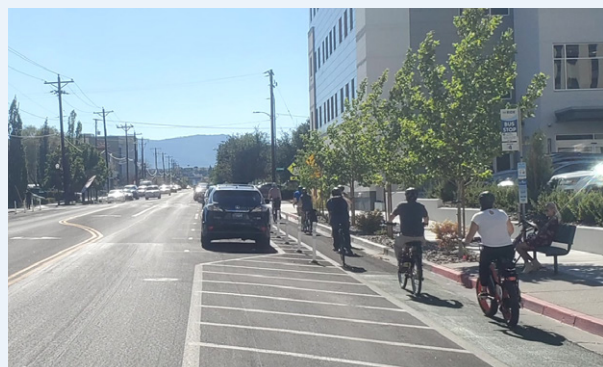
The recent quick build project on 5th St (above) in Reno helped the RTC test the parking protected bike lane design
