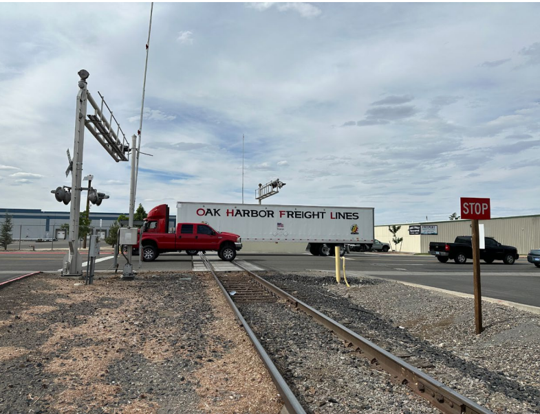
Existing rail spur crossing Glendale Avenue
