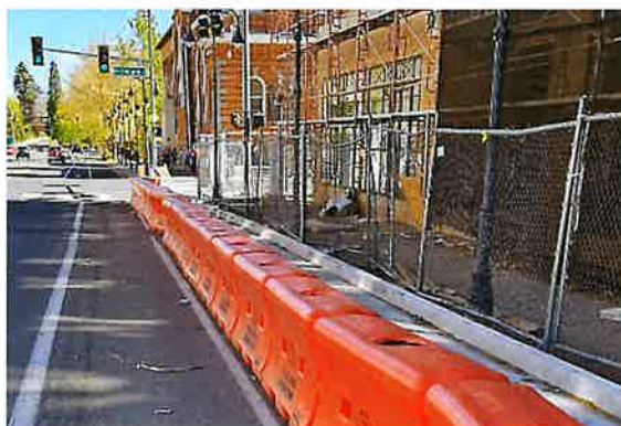
Figure 6.6 Water-filled barriers on Arlington Ave which can be used for quick-build installations.
