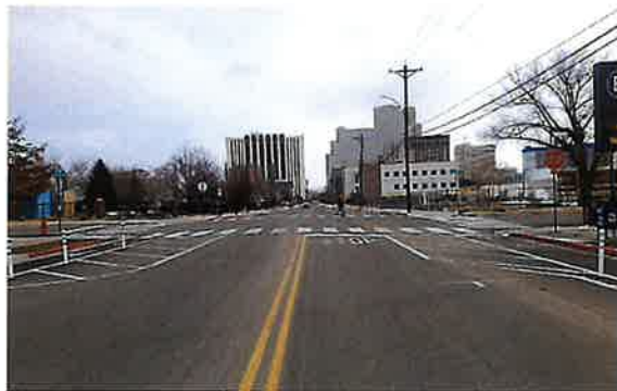
The 5th Street project is an example of local quick-build project implementation.
