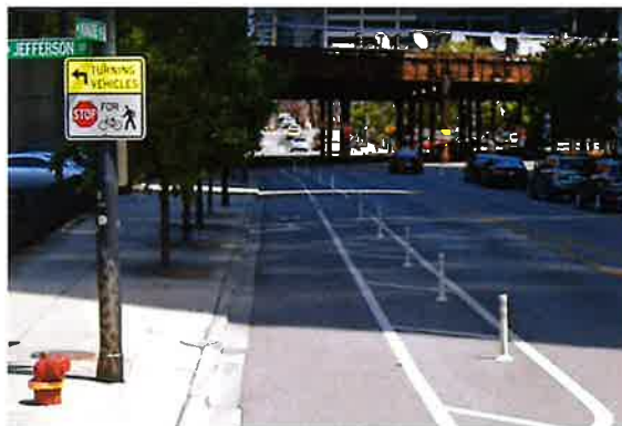
Figure 6.4 Vertical Buffer Alignment Placement to Accommodate Wide Bikeway Sweepers (Source: Google (Imagery - August 2019), W. Kinzie Street looking east at N. Jefferson Street).
