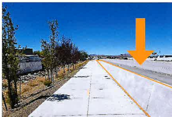
Figure 6.5 Concrete barrier between shared-use path and vehicle traffic on Sparks Blvd.
