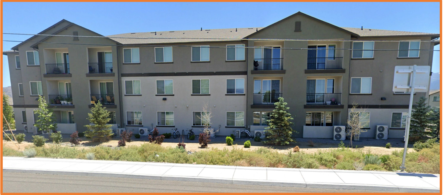
Steamboat Apartments Located Along Geiger Grade (SR 341)
