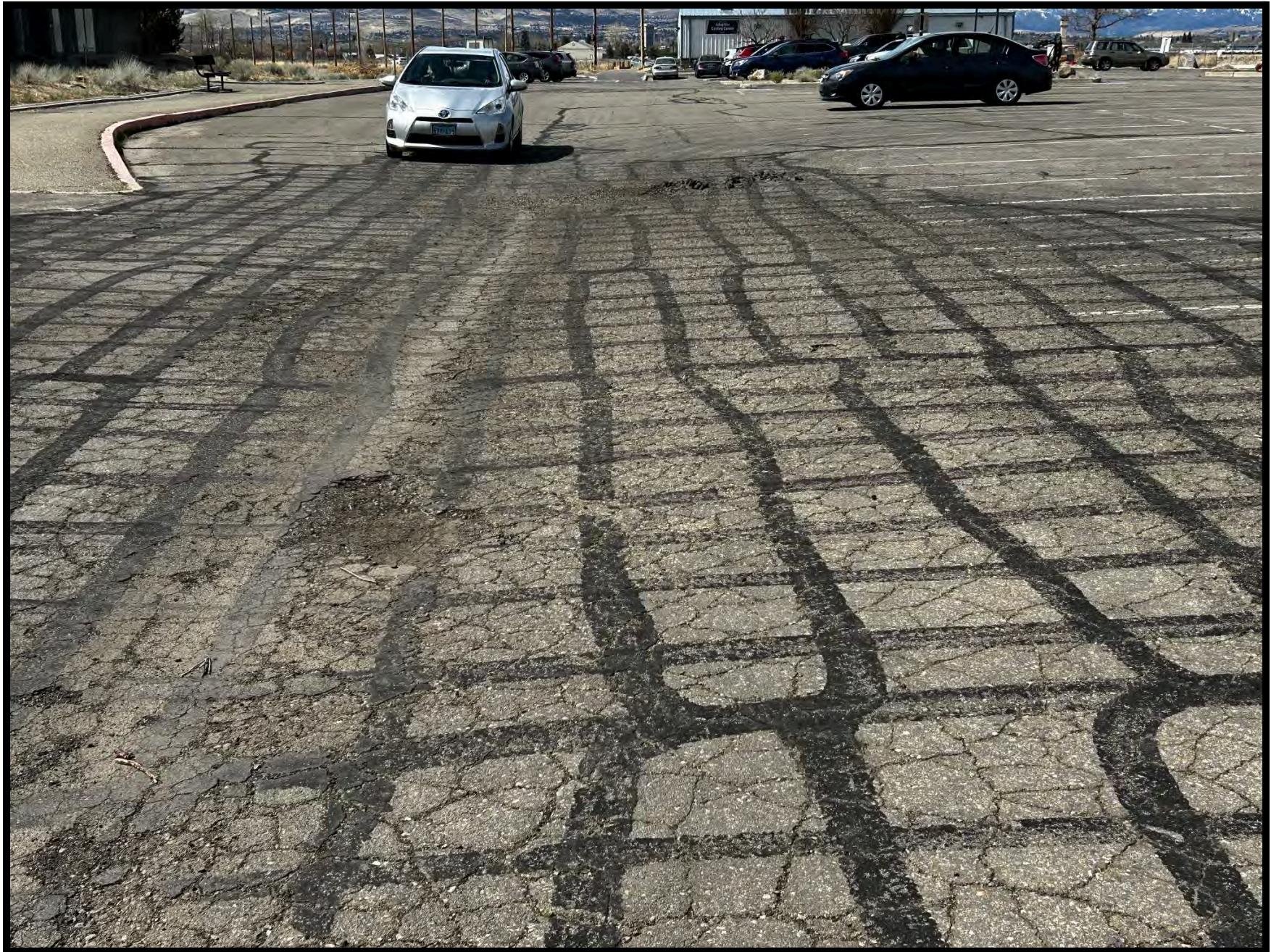
Rosewood Parking Lot Failure - covering most of the parking lot_March 2025
