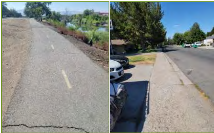
Figure 10-Path Width Examples (Meets Recommendation / Does Not Meet Recommendation)
