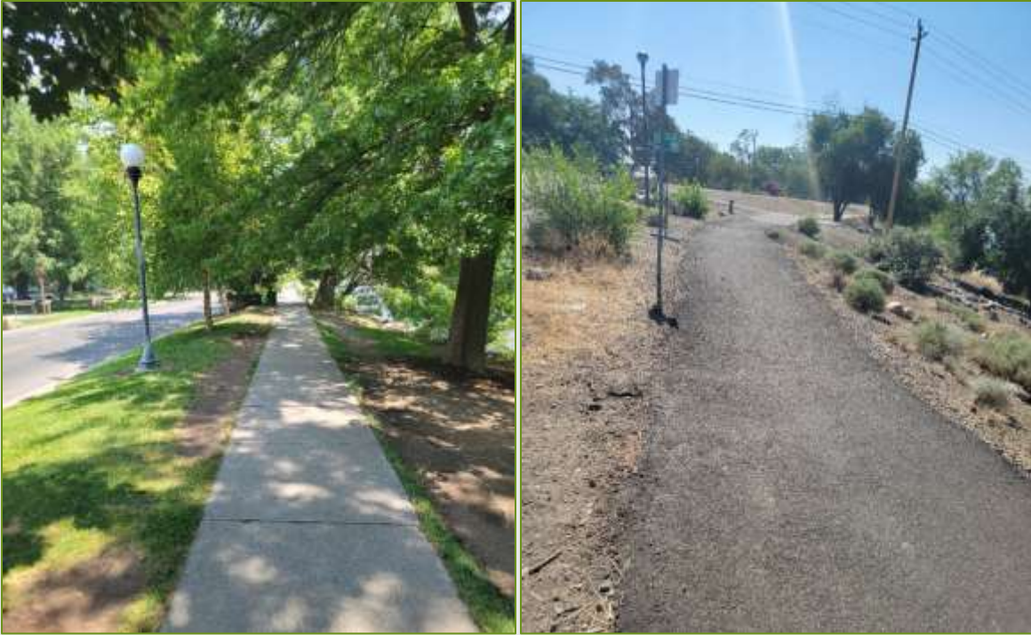
Figure 15-Longitudinal Slope Examples: Concrete Within Recommended Slope / Asphalt Outside Recommended Threshold)
