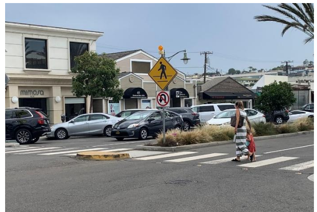
Figure 14. Pedestrian Median Refuge Island Example
