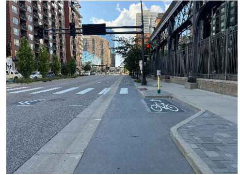
Figure 12. Bicycle Jug Handle Example
