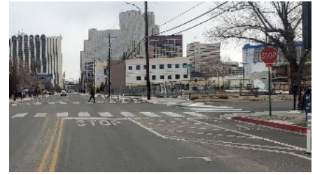
Figure 8. Quick-Build Curb Extensions Example
